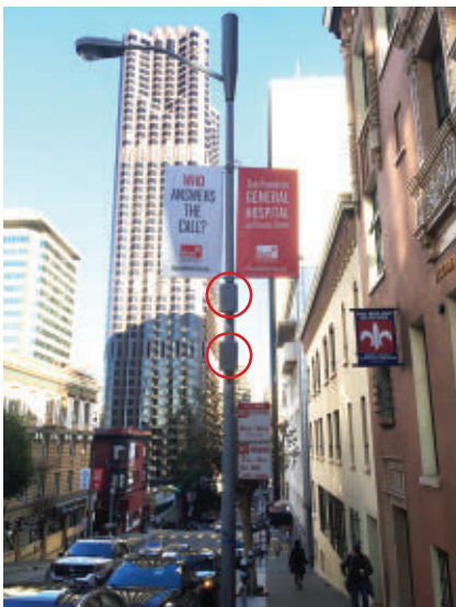
▲ Fig. 3 Ericsson microcells for Bands 2 and 4, deployed on a streetlight in San Francisco, Calif. Source: ETL Wireless.
